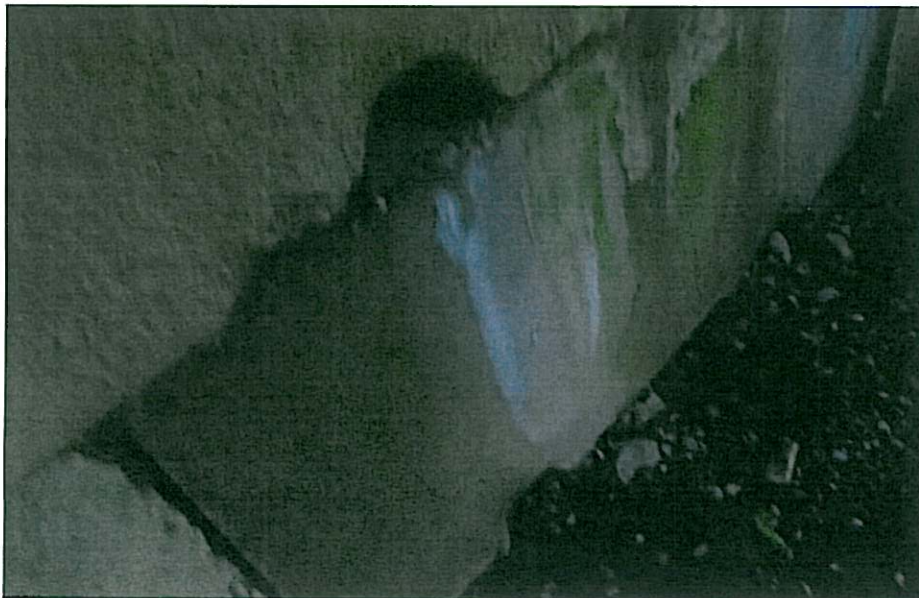
CK-2390 Left abutment 2
