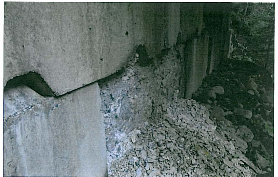
CK-2390 Right abutment 1
