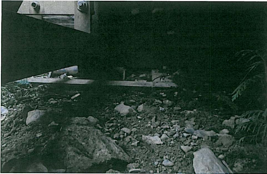
CK-2390 Right abutment 2
